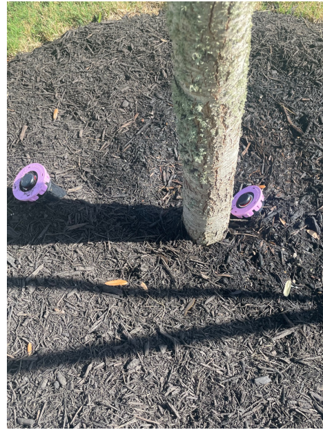
Bubblers too close together
