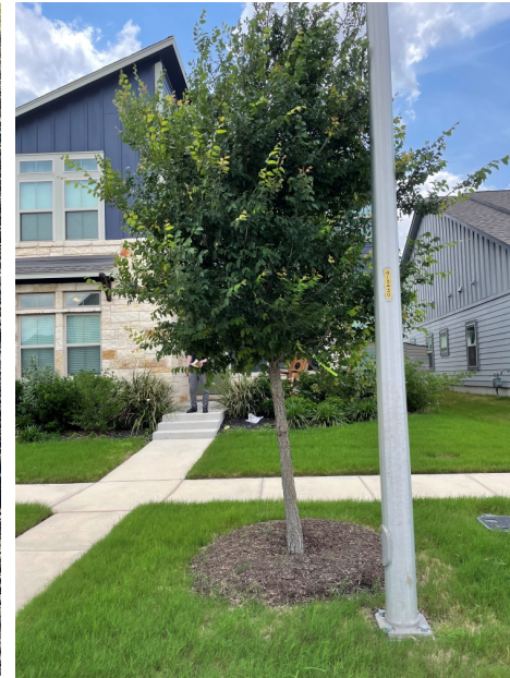
Tree installed too close to light post
